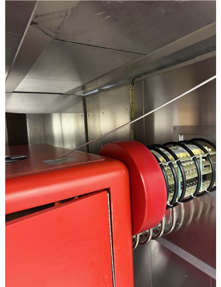
Enclosure internal lead shielding and grounding drop bars were removed (2)
