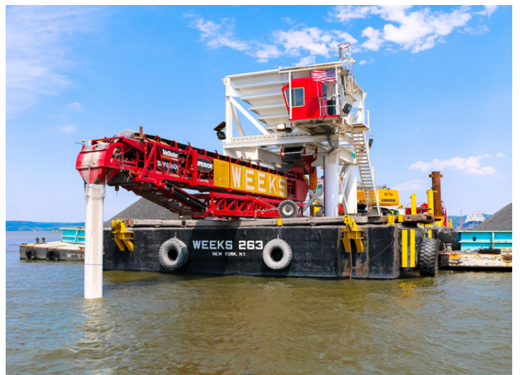
BARGE UNLOADING / DREDGE CAPPING
